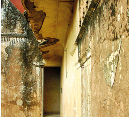
Deteriorated condition of Chajias/overhang
