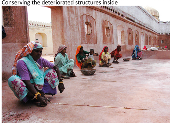
Process of doing the lime flooring
