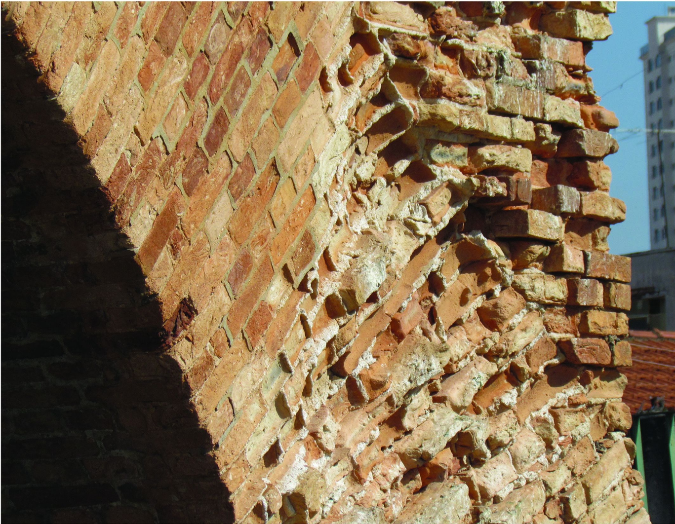
Bricks with loss of mass
