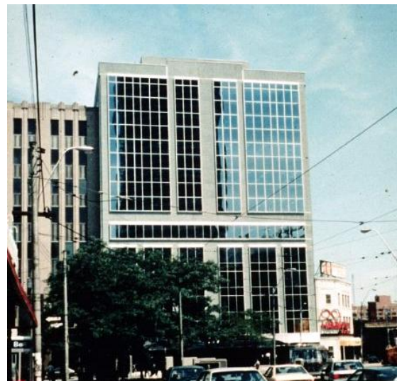
Fig. 5b – The final facade after super elevation, where the distinction between the old and the new parts is clearly identified
