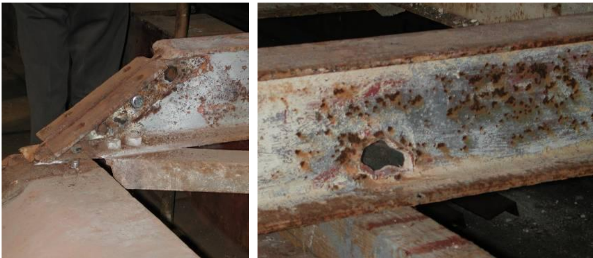
Figure 9: Details of the state of deterioration of the various steel elements. Various sections of the bridge were also damaged with shrapnel that punctured the web.
