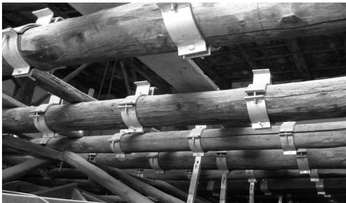
Figure 16. Consolidation intervention on the wooden floor structure in the Diplomatic Hall of the Royal Palace of Naples.
