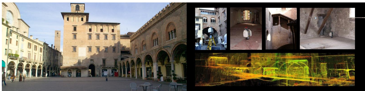
Figure2. View of the Mayor's Palace (Palazzo del Podestà) from Piazza delleErbe Phases of indoor metric acquisition with Leica Laser 3D HDS 3000
