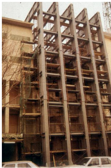
Fig. 6a – New extension, both vertical and lateral, in the Jolly Hotel in Caserta, with three additional floors.
