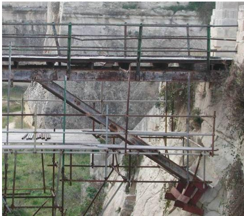
Figure 6: photograph showing the previous 'repairs' on the bridge: the rudimentary angle iron railing uprights; the series of transverse beams that supported the metal sheeting deck; and steel corbels beneath the original abutments.
