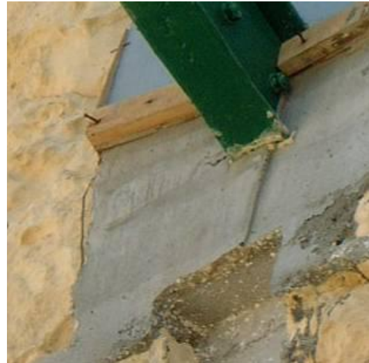
Figure 14: Detail of grouting of the resulting holes from the removal of the steel corbels. Grouting was left short of the rock face to allow application of hydraulic lime mix to achieve original abutment detail
