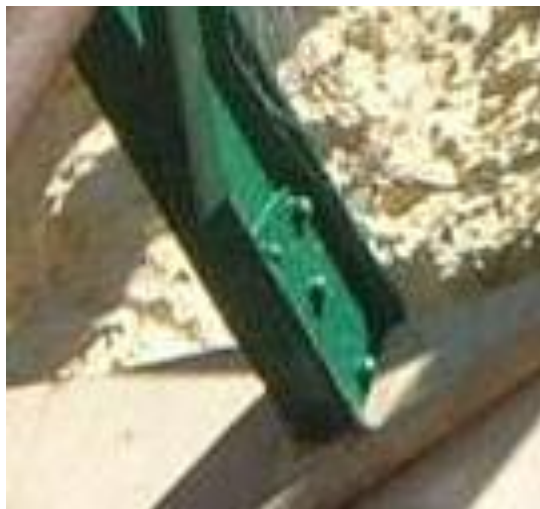
Figure 15: Detail of the repair plates at the ends of one of the inclined struts.
