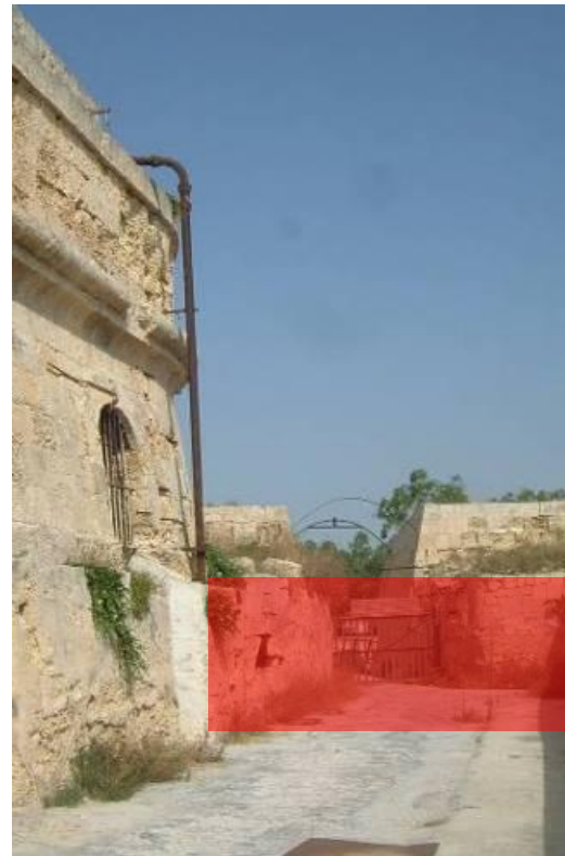
Figure 3: A photograph of the area showing the extents of the drastic alterations in the original floor level of the Fort to allow 'vehicular' access into the Fort.
