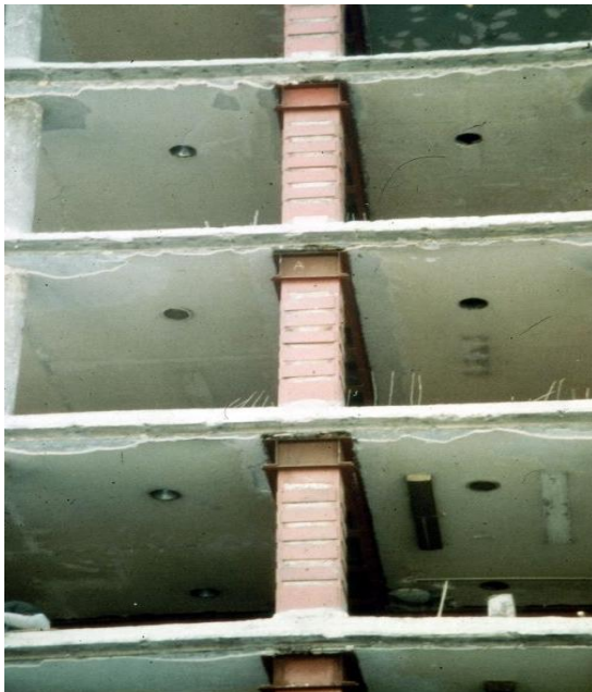
Fig. 14 – Steel angles in the corners and transversal batten plates for strengthening r.c. columns in Mexico City.
