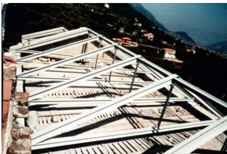
Fig. 7 – A new steel structure for roofing a church, substituting the old one ( lightening ).
