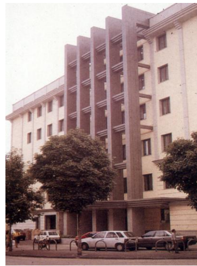
Fig. 6b –The new facade of the Jolly Hotel in Caserta, which has been aesthetically improved by the presence of steel portals.
