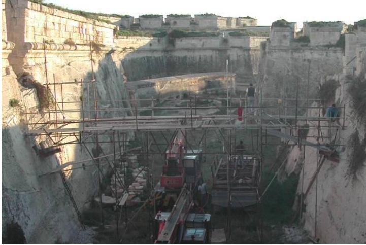
Figure 8: View of the ditch after the bridge was dismantled and the last section loaded on the trucks to be taken to the workshop.
