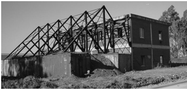
Figure 4. The real reinforced concrete building in Bagnoli, cyclically tested until collapse and then repaired by means of different techniques.
