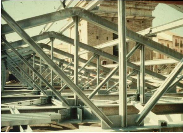
Fig. 15 – A new steel truss as a roof in the structural restoration of a church.
