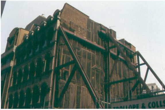
Fig. 1 – Temporary steelworks used in rehabilitation operations ( safeguard ).
