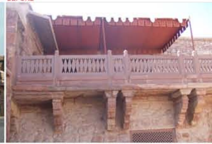
HAVELI - J, WITH NEWLY CONSTRUCTED STONE RAILING - AFTER
