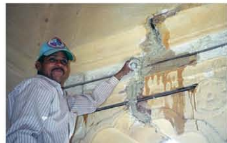
REPLACING IRON CLAMP BY STAINLESS STEEL ROD STITCHING
